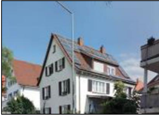
Abb. 27: Schleppgaube
