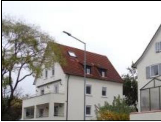
Abb. 25: Schleppgaube
