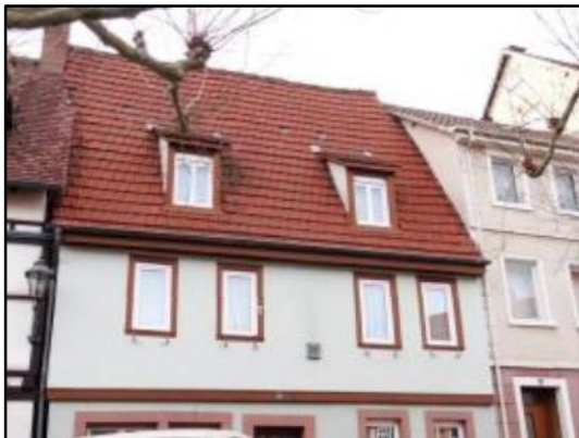
Abb. 20: Schleppgaube
