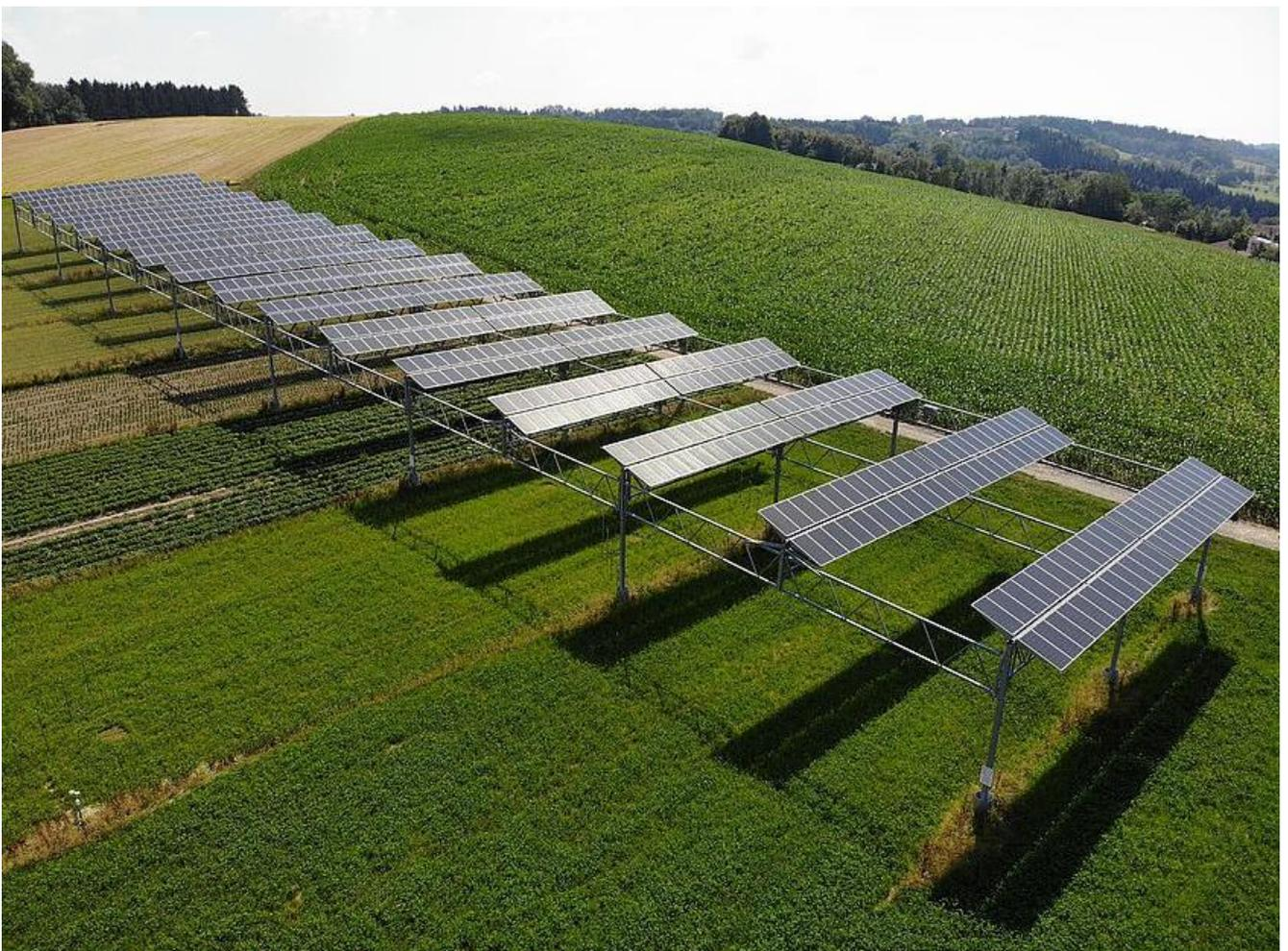
**Abb. 2: Agri-Photovoltaik in Heggelbach am Bodensee, Fraunhofer ISE**
